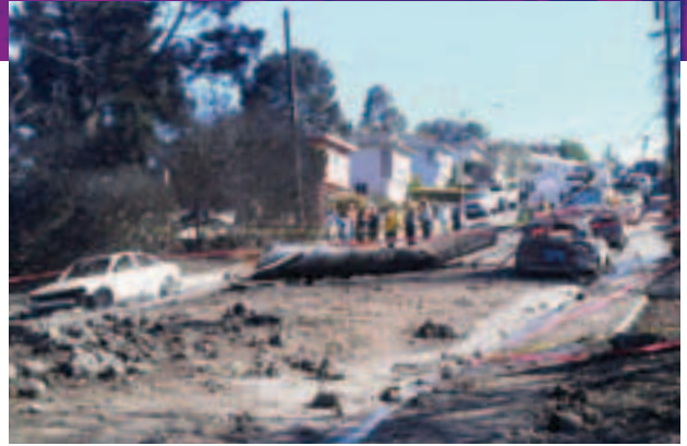
A repair project at a Pacific Gas and Electric facility went awry just before the San Bruno pipeline explosion in California last September. Both lives and homes were lost as a result.
